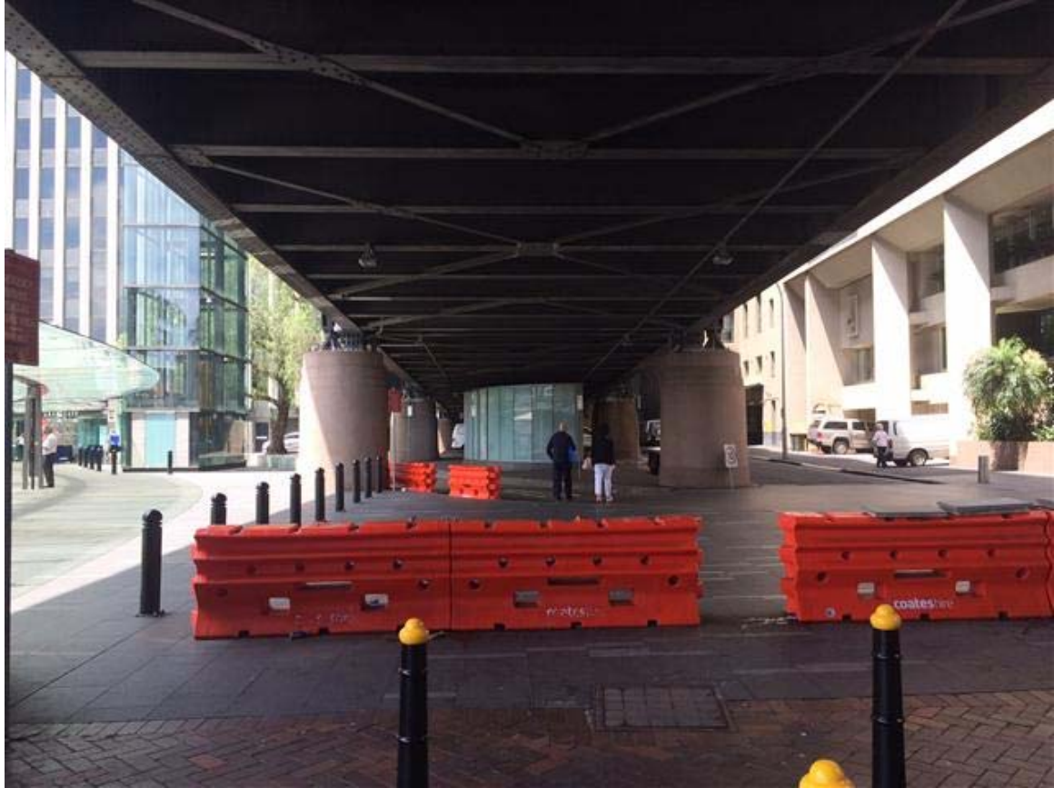
Figure 14: Existing access road and underpass below viaduct and RMS amenities building.
