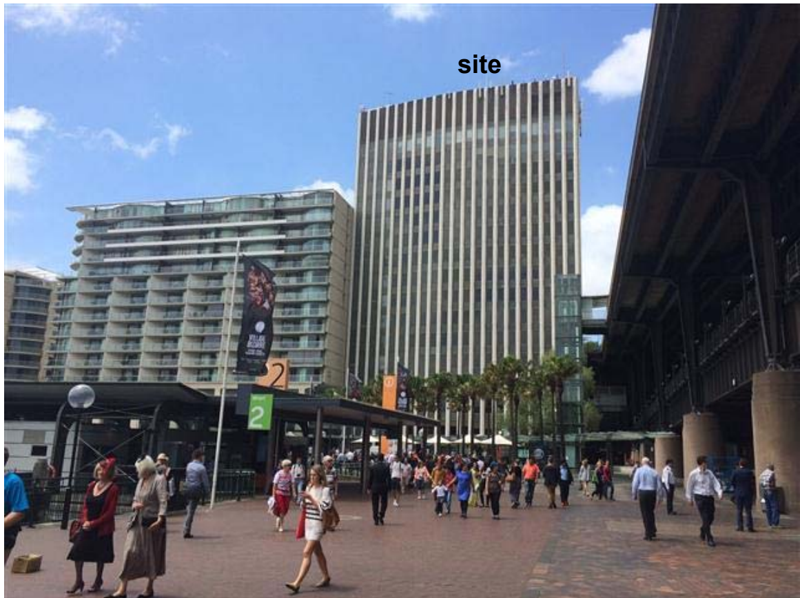
Figure 3: The Site, as viewed from Circular Quay in an easterly direction.
