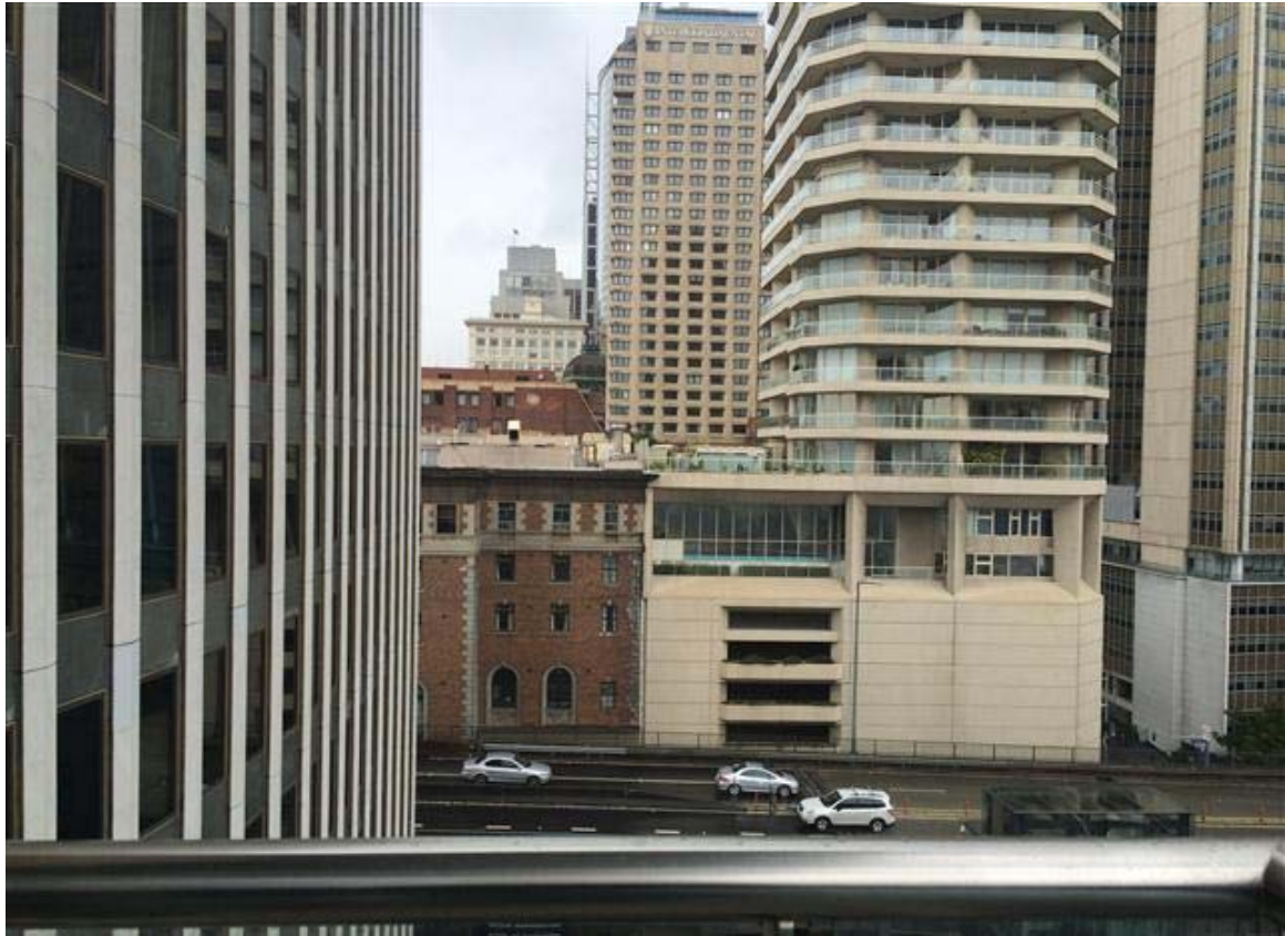
Figure 45: Photograph taken from Quay Grand balcony looking directly south over the subject site towards CBD.
