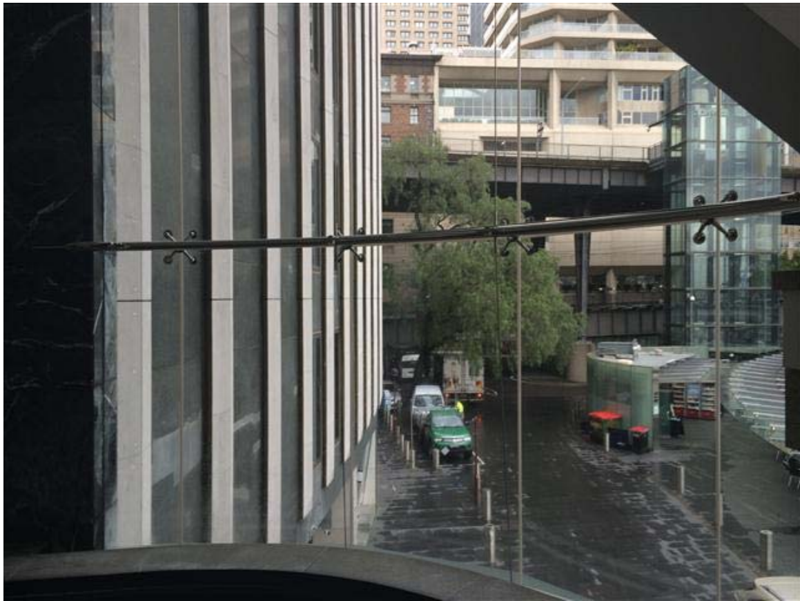
Figure 7: Elevated view of the existing vehicular access road from Level 2 of building to the north of the site.
