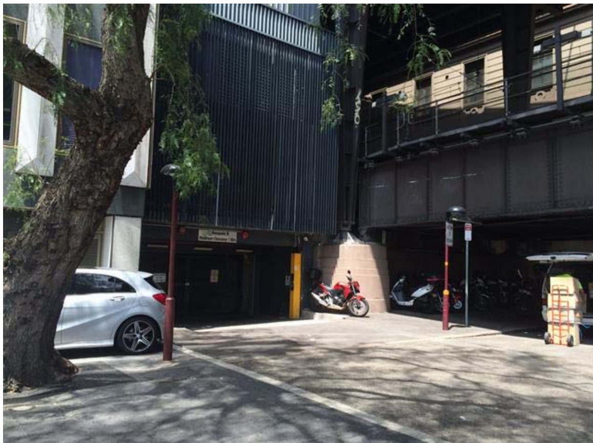
Figure 6: Existing vehicular entry to the building adjacent to the rail viaduct.
